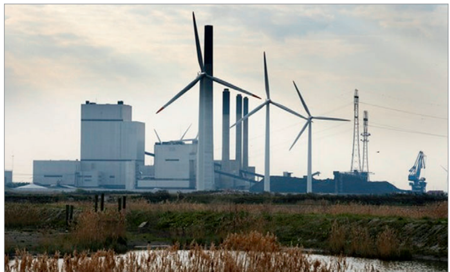
Figure 9.3: Nordjyllandsvæket USC combined heat and power plant [Source: Vattenfall]
