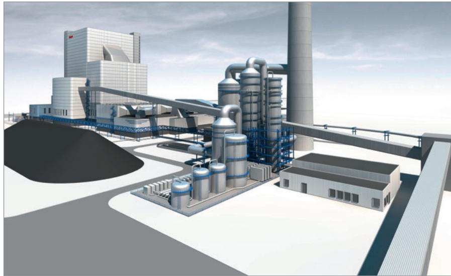
Figure 8.1: Schematic impression of the 250 MW e capture unit (post-combustion) at the ROAD project in Rotterdam, the Netherlands [Source: ROAD / Global CCS Institute]
