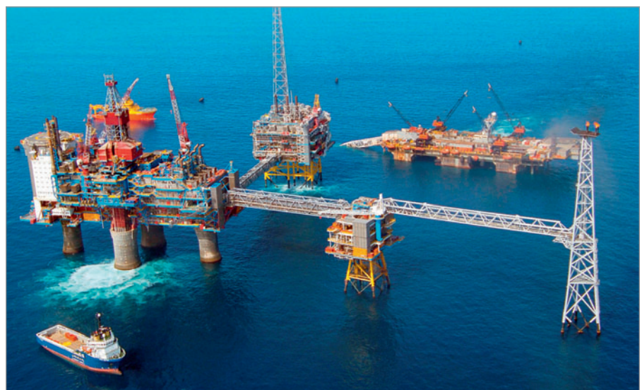
Figure 8.2: CO 2 capture and injection at Sleipner (Norway) [Source: Klm Laland/ Statoil]
